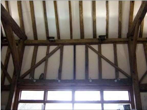
this is where the top of the threshing doors were. Mortises set on the 'door' side of the adjacent roof beams would tend to confirm this as it was customary to place roof braces on the door-side of the posts nearest the opening. The northwest corner has a good example of a root stock upright post. Placing the tree-trunk upside-down allows the top to splay out and provide enough material for the complex jointing needed.
